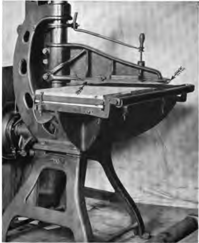
Fig. 3. Clicking Machine equipped with Finger Guard.*
